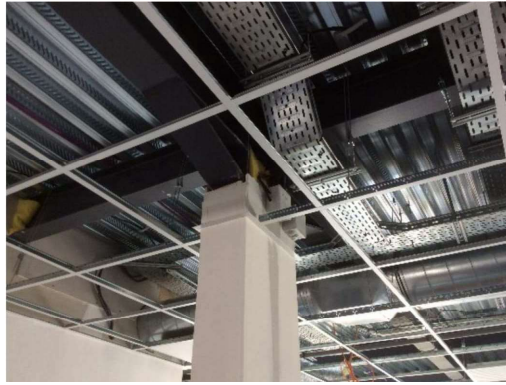
Illustration 13 : a detour of the ventilation duct had to be realized on site
