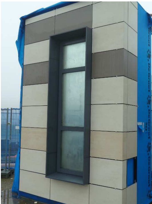
Mockup façade for airtightness test
